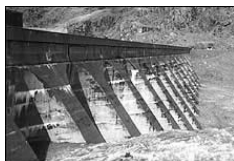
Photo: Stwain Dam in Wales http://www.britishdams.org/about_dams/butress.htm
