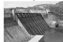
Photo: David Brodbeck, Grand Coulee Dam Spillway
