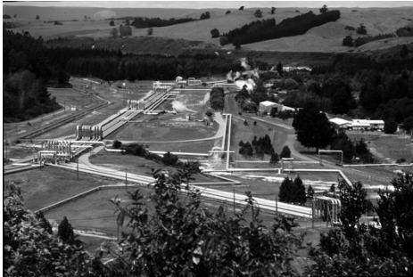
Ohaaki Geothermal Power Station, New Zealand
